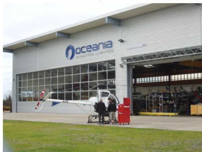
The first 2 TRU-FOLD™ doors installed at Ardmore airport.
